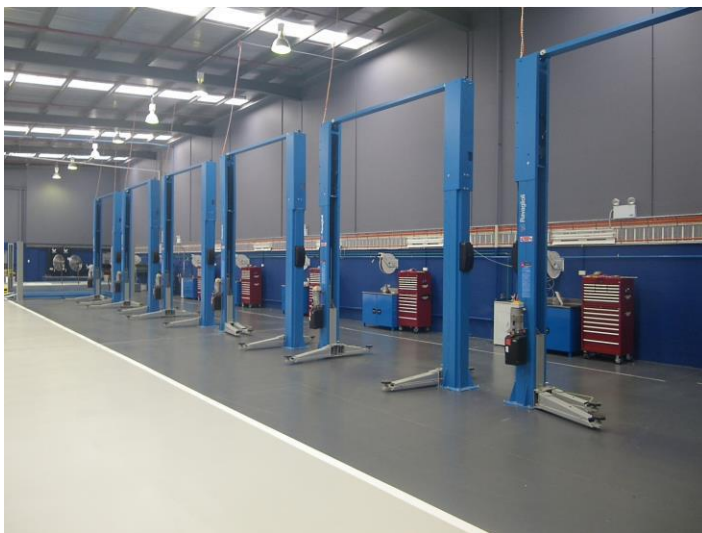
Minc Services Project: Shop Fit Out
