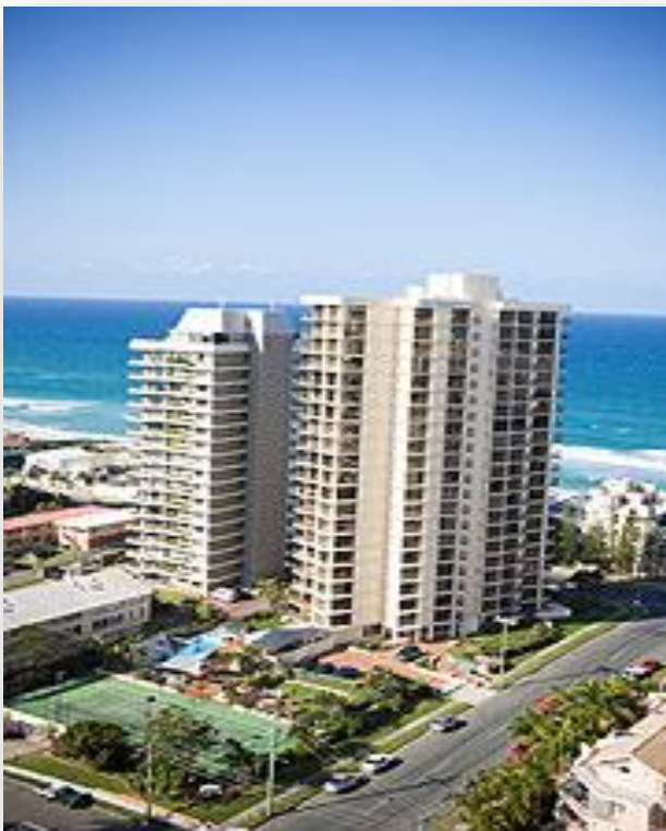
Minc Services Project: Remedial repairs to entire building exterior and full exterior repaint
