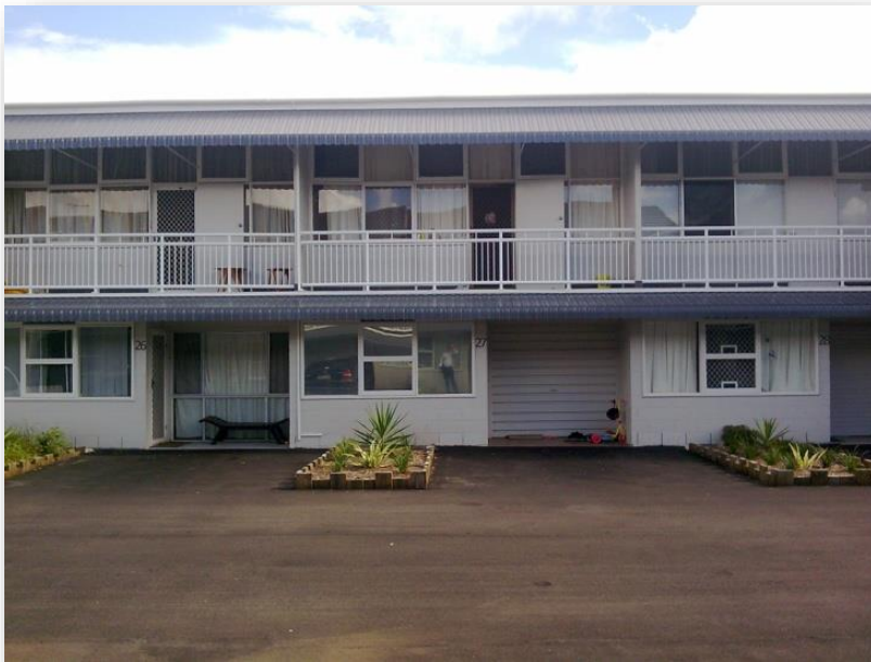
Minc Services Project: Concrete Works
