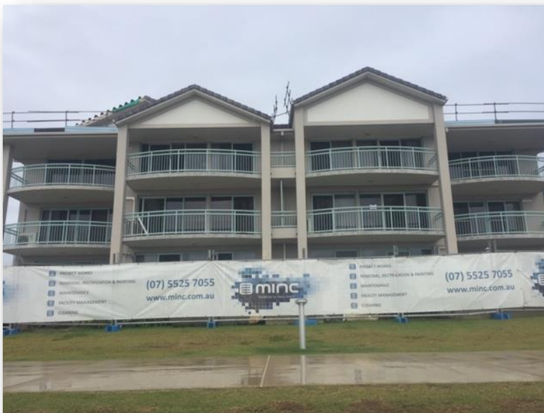
Minc Services Project: Roof Replacement – Waterproofing - Repaint
