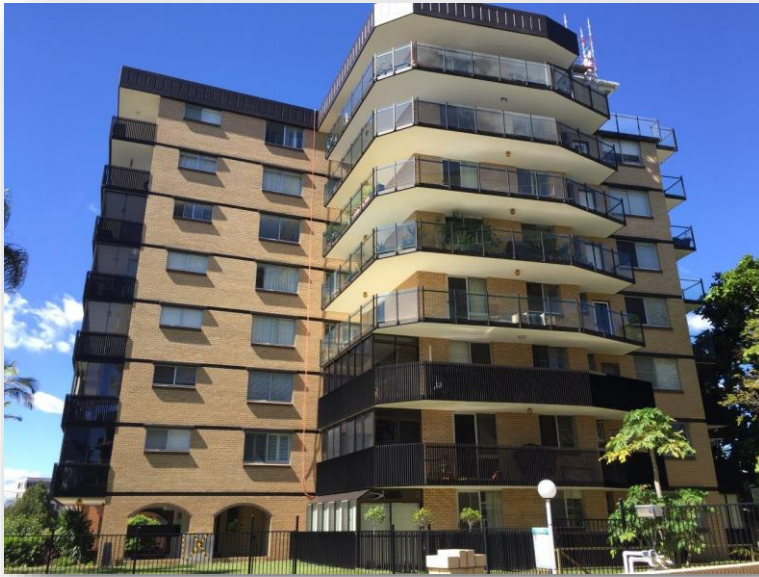
Minc Services Project: Remedial repairs to entire building exterior
