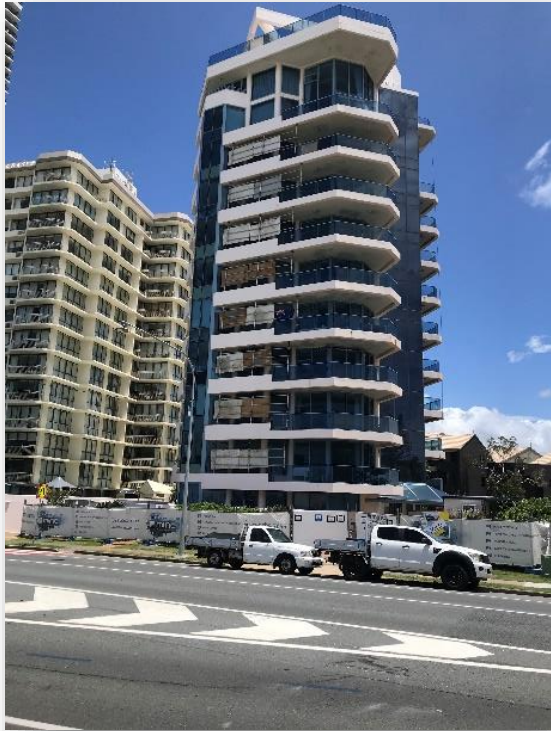
Minc Services Project: Building upgrade, and refurbishment work
