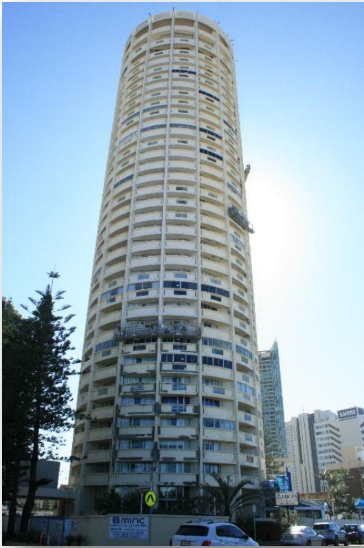
Minc Services Project: High Rise Re-paint
