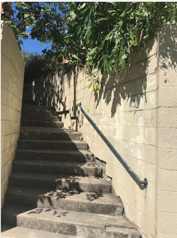
Minc Services Project: Public Staircase Replacement
